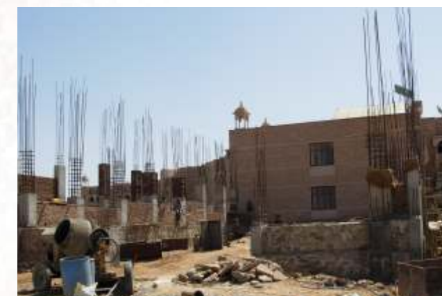
Conference hall work progress
