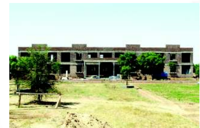
Scientist training hostel work progress
